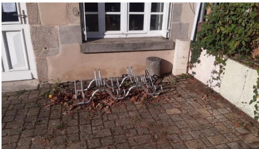
FIGURE 21 SYSTEME DE PINCE ROUE, A EVITER
